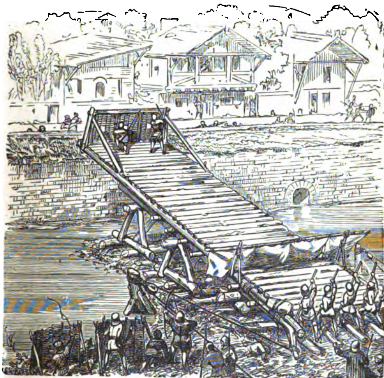
FIG. 26.—THE ATTACK—THE MOVABLE BRIDGE INTENDED FOR CROSSING THE SMALL ARM OF THE RIVER OF AROBIA.
